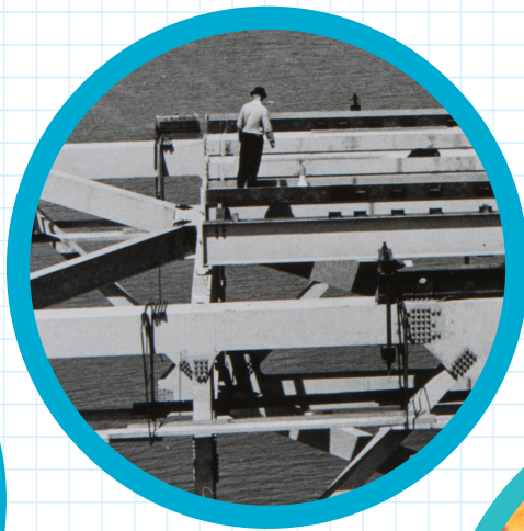
○ Raising the trusses on the Tamar Bridge
